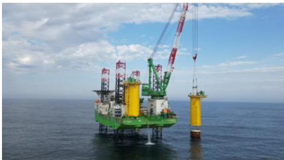
c) Moray West transition piece installation by Apollo
