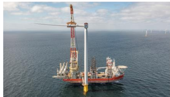
f) Moray West blade installation by Wind Orca
