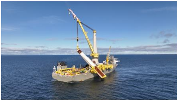
b) Moray West monopile installation by Bokalift 2
