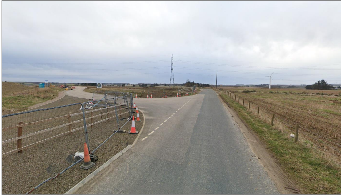
Photo 2: Proposed location of Substation Site construction access (unclassified road, looking north) Source: Google
