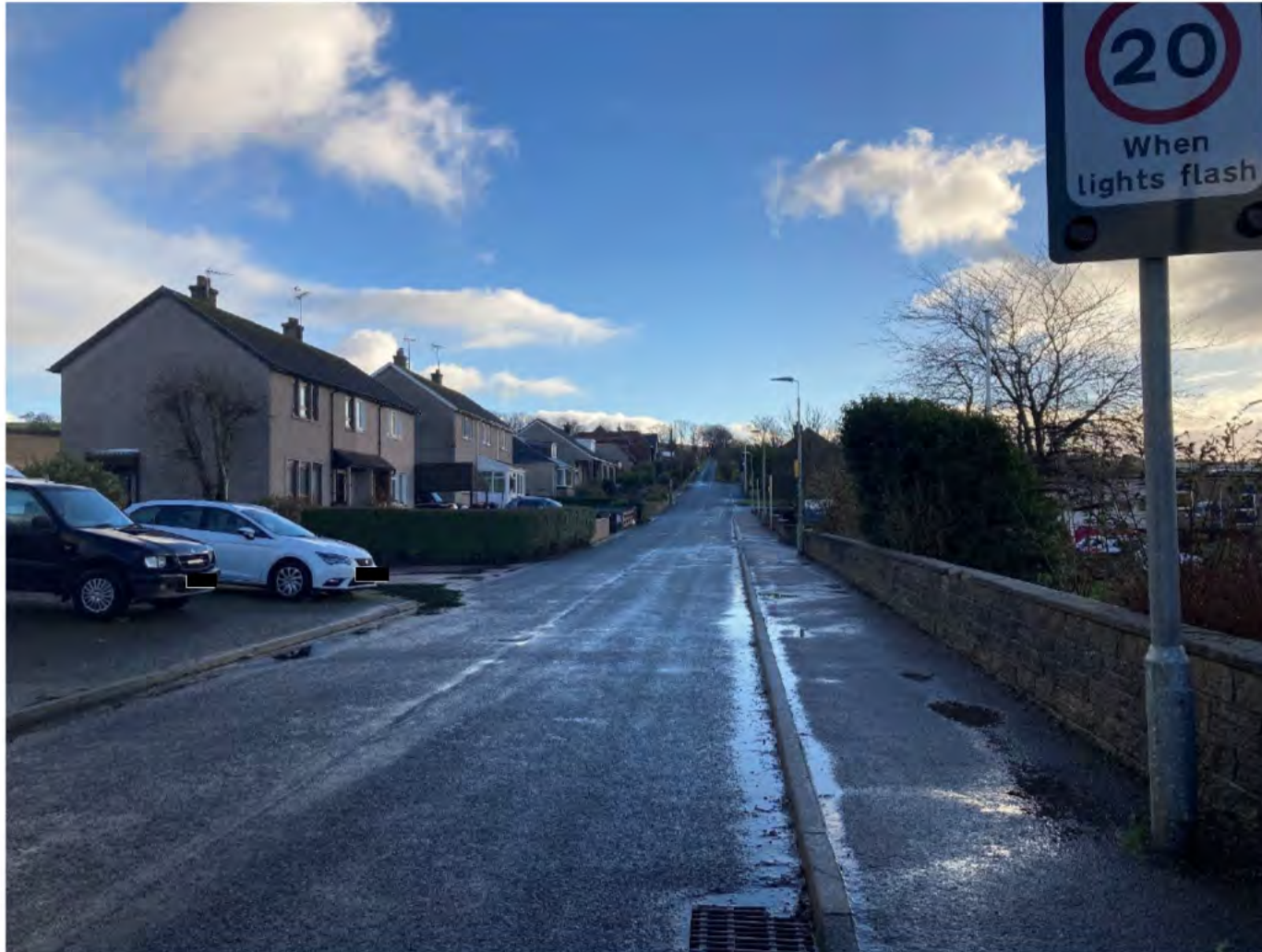
Plate 6: View along Thornhill Road towards ridge bordering Cuminestown to the south facing south/south-east
