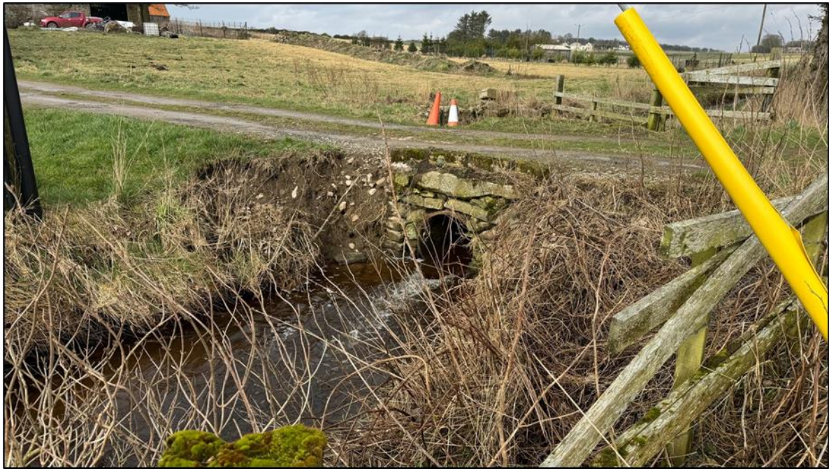
Photograph 30: Burn of Asleid (WC13), Culvert.
