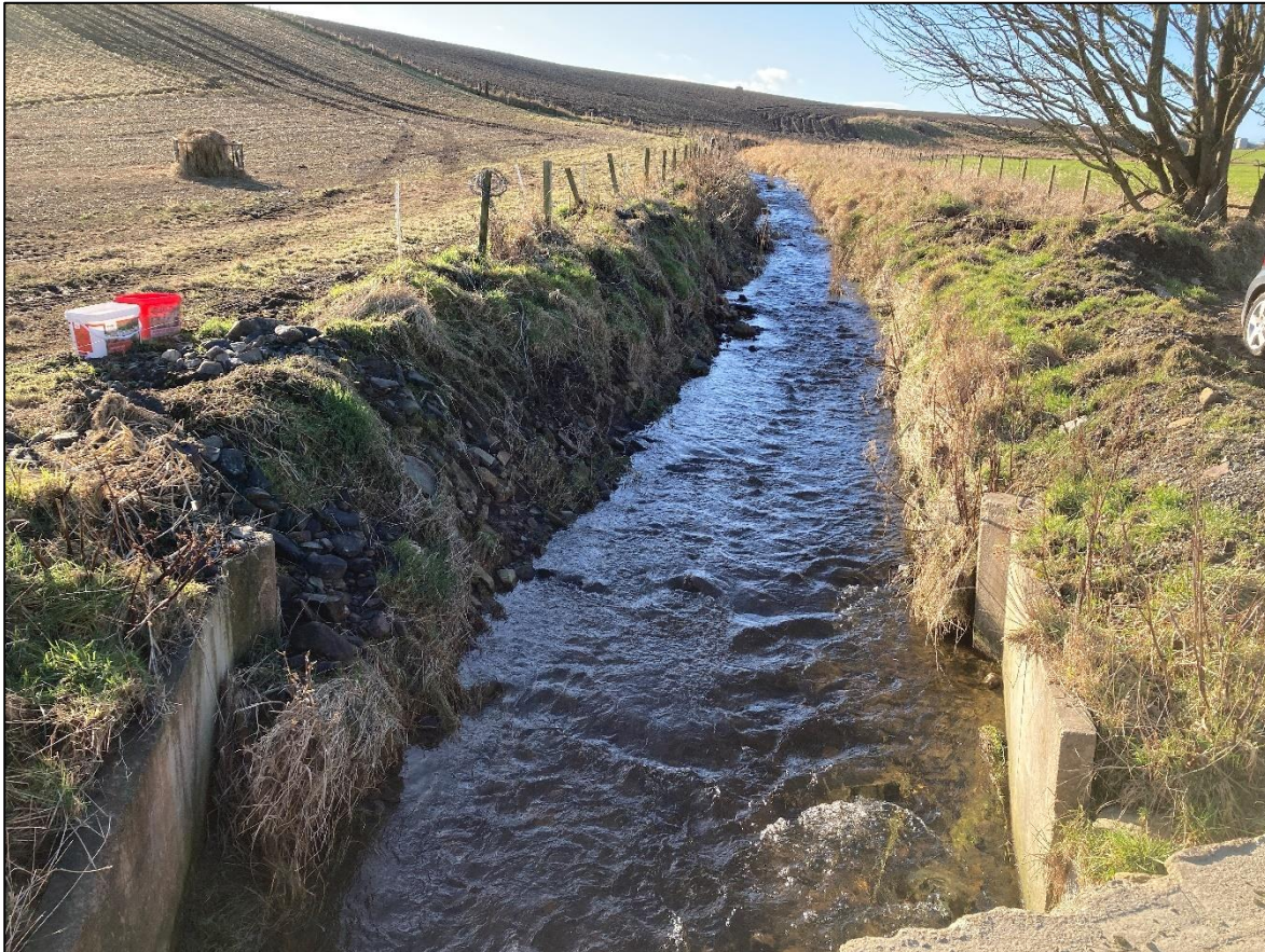
Photograph 6: Burn of Brydock (WC03), Widened and Embanked Section of Channel.
