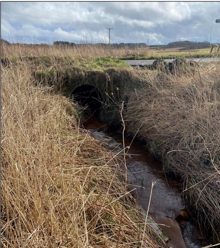
Photograph 28: Burn of Balquholly (WC12), Culvert under Minor Road.
