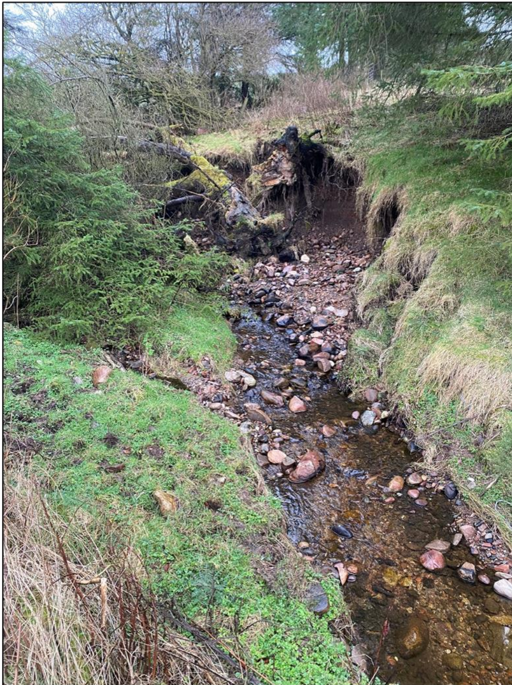
Photograph 24: Glen Burn (WC11), Erosion and Overhanging Trees.
