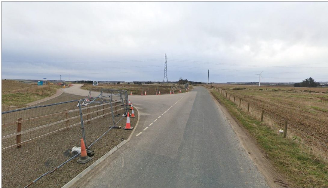
Photo 1: Proposed location of Substation Site construction access (unclassified road, looking north) Source: Google
